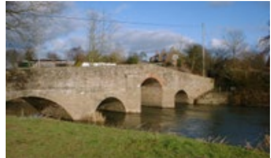
Laystone Bridge - a grade 2* listed structure
