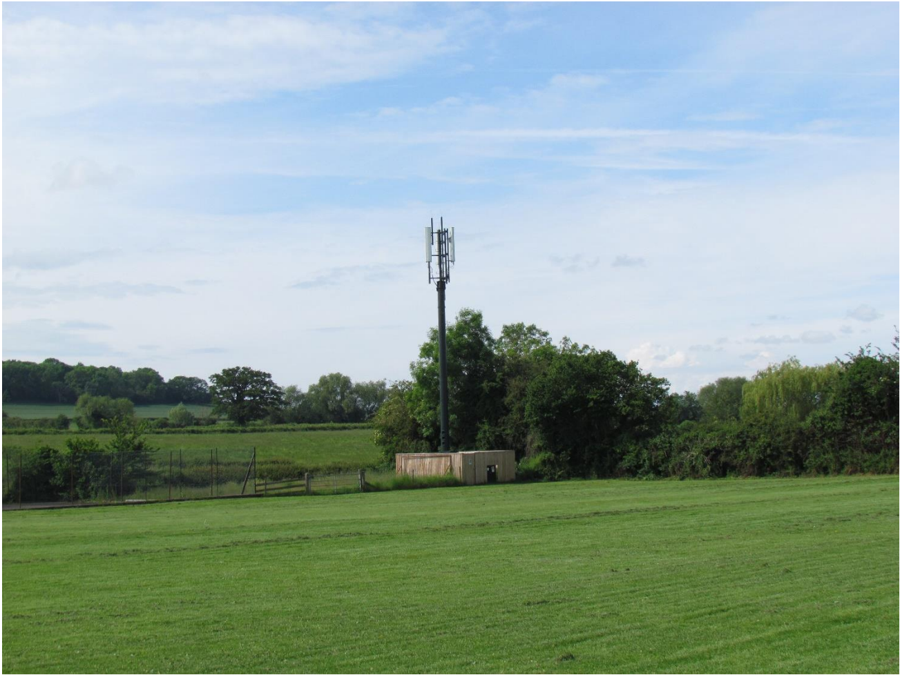
Figure 2 – Marden Recreation Ground Radio Base Station Site
